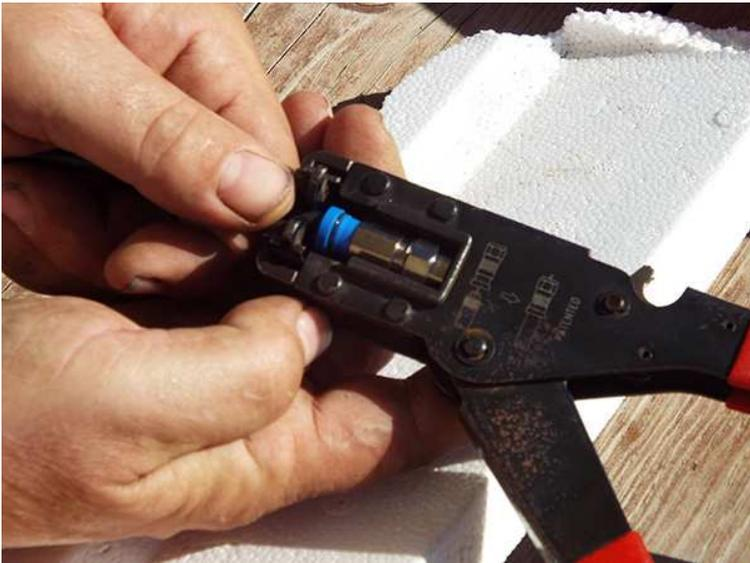
Push the connector firmly into the tool.
