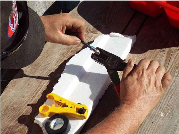
Remove the completed connector/cable at an angle as it was installed.
