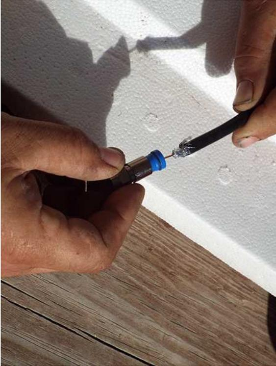
Slide the connector onto the coax carefully aligning the center conductor.
